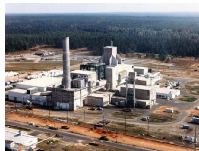
L Reactor at SRS
