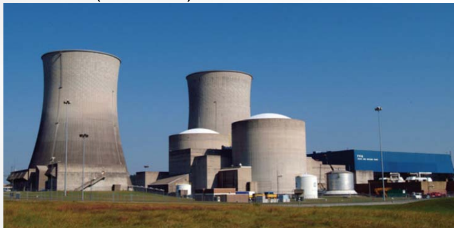
Watts Bar Nuclear Plant Spring City, TN
